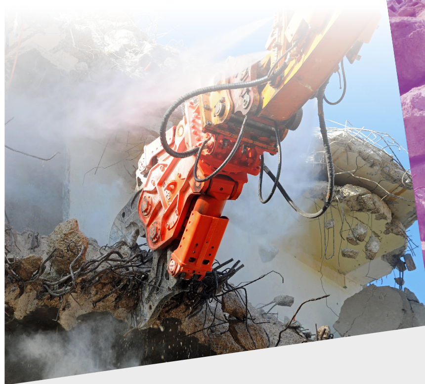
▲ Demolition by pliers
