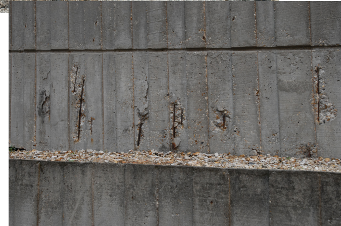
▲ Example pathologies (spalling) of reinforced concrete due to reinforcement corrosion induced by carbonation.
