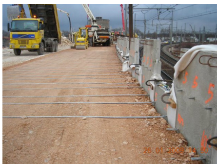
▲ Retaining wall next to the track
