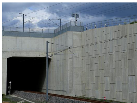
▲ Retaining wall on SEA HSL 3
